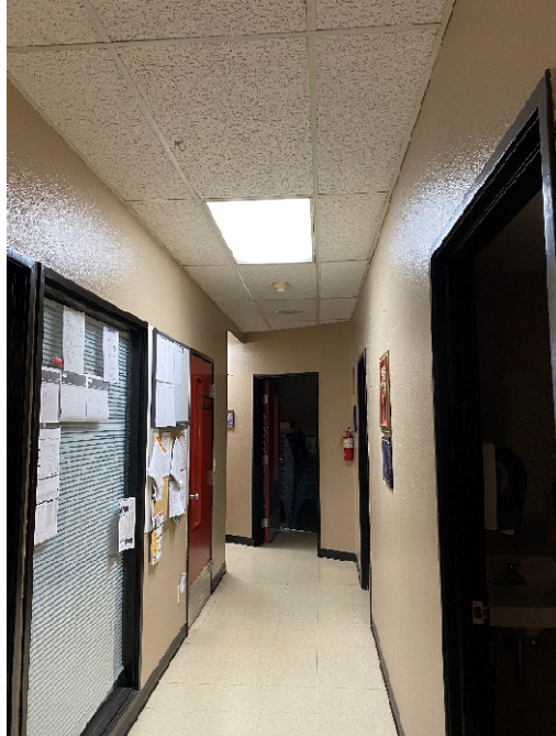
Image 6: Interior Corridor Ceiling
