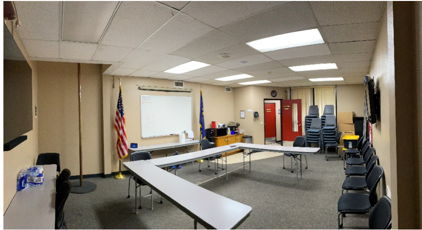
Image 7: Interior Board Room Ceiling
